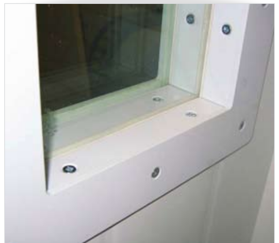
Steel frame of high security window.
